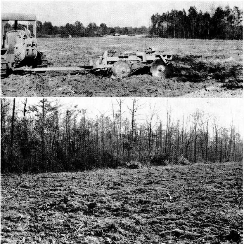
FIGURE 8. (Above) Type of plowing harrow used on experimental plots after disposal of material in windrows was completed; (below) condition of land after plowing plot cleared with KG blade on D-6 tractor.
