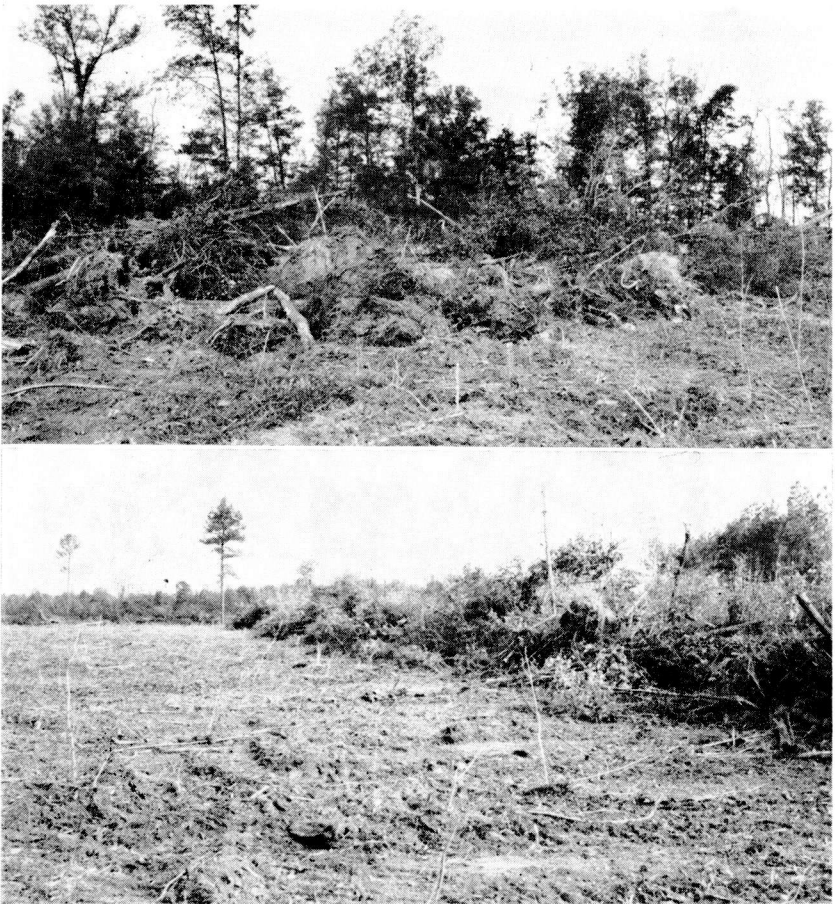
FIGURE 5. (Above) Windrow made with bulldozer blade, and (below) windrow made with KG blade.
