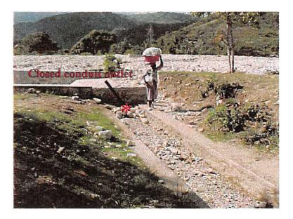
Photo 14. Sediments and gravel filled main canal at the closed conduit outlet.
