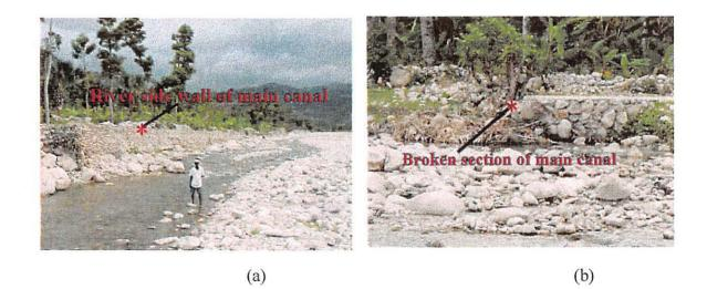
Photo 4. Upper section of main canal at Belle Roche below the intake structure has survived due to the rock wall structure, but the lower part of this section has been broken as shown in the right photo.
