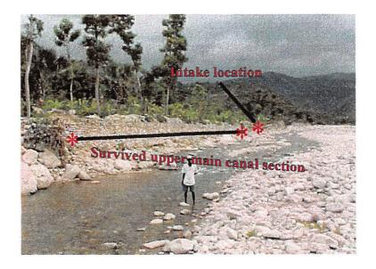
Photo 10. Damaged upper section of main canal at the Belle Roche site. The rock walled section of the main canal survived the flooding but the left end of the section was completely cut off.
