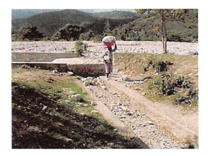
Photo 8. Sediments completely filled up the main canal at the outlet site of the closed conduit. This was caused mainly by the flooding.
