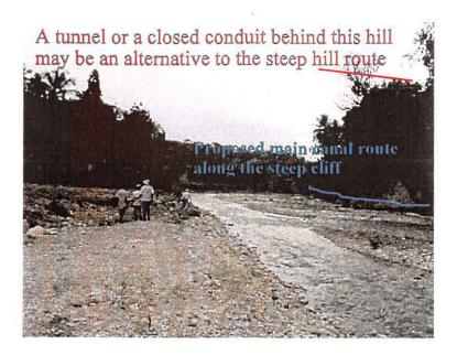
Photo 24. A steep cliff on the west bank will be a difficult task to route the main canal as proposed. An alternative would be to install a closed conduit or a tunnel behind the hill. This section of the proposed main canal is relatively short.
