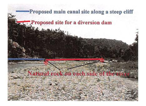
Photo 25 Proposed intake and upper section of the main canal route.
