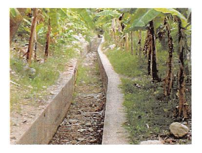
Photo 6. Undamaged section of main canal. Except for the upstream section the main canal below the siphon structure survived the hurricane George. Sedimentation and trash accumulation were excessive which would cause serious problems if not adequately cleaned up.
