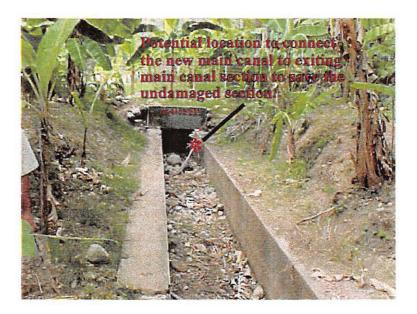
Photo 16. Potential site to connect the new main canal to exiting main canal to save the existing main canal and the closed conduit.
