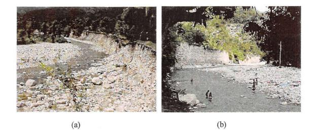
Photo 17. Severe bank erosion which destroyed the road and canal. Left: from downstream side. Right: from upstream side. A drastic river course change is required to prevent further bank erosion.
