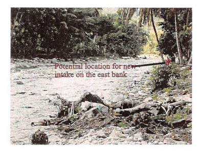
Photo 11. Potential location of a new intake site on the east bank of the river to avoid a river crossing structure. Location is determined by the elevation change in the river which should be high enough for gravity supply to the undamaged section of the main canal. The new connecting section may be routed near the foothill to avoid future damage by flooding or bank erosion.
