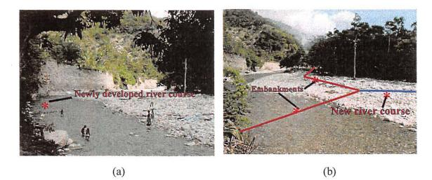
Photo 20. The flooding caused bank erosion and changes the river course further inland while depositing more sediments on the right side of the flow. Stabilization of the bank and change of the river course is necessary to protect the hillside. (b) shows approximate location of embankments and new river course open.
