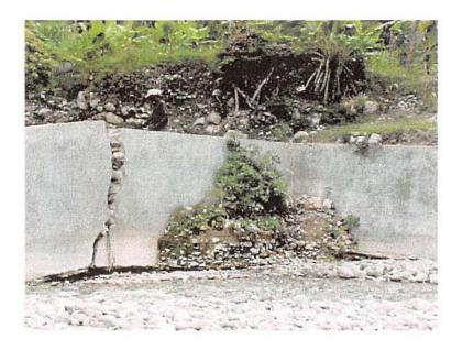
Photo 2. Intake structure at Belle Roche site. Note the broken left wing. The intake sluice gate locates behind the wall covered with grass.
