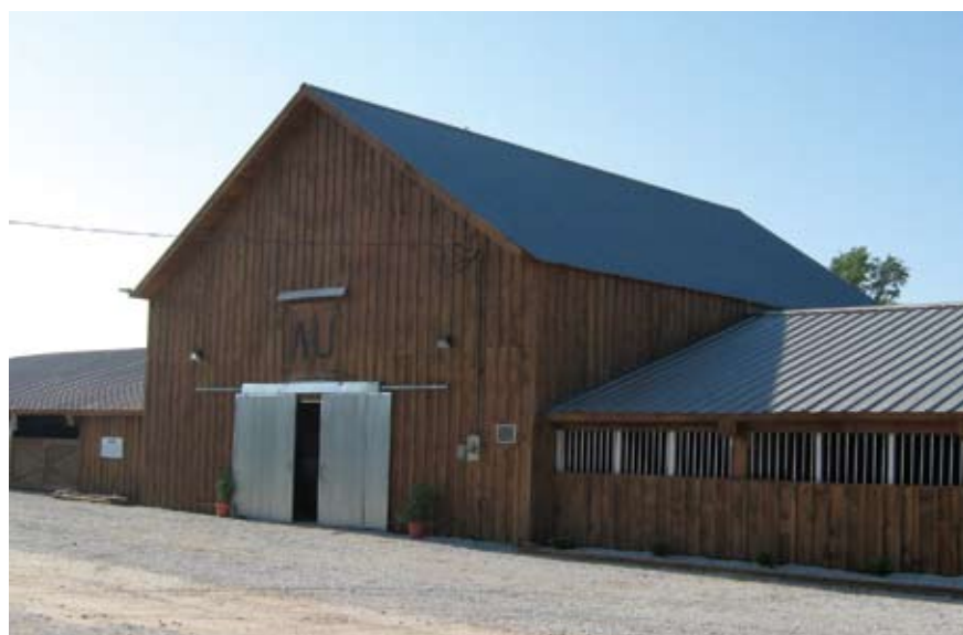
FACELIFT COMPLETE —The barn at the AU Horse Unit has had a new facelift that gives it the look of an old-fashioned board-and-batten barn, thanks to the work of the AAES Agricultural Land and Resource Management team.
