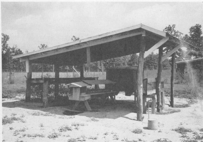
House No. 5. — Roof only; all four sides open.
