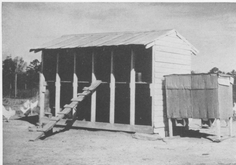
House No. 9. — Only roosts are protected with tight north, east, and west walls and roof.
