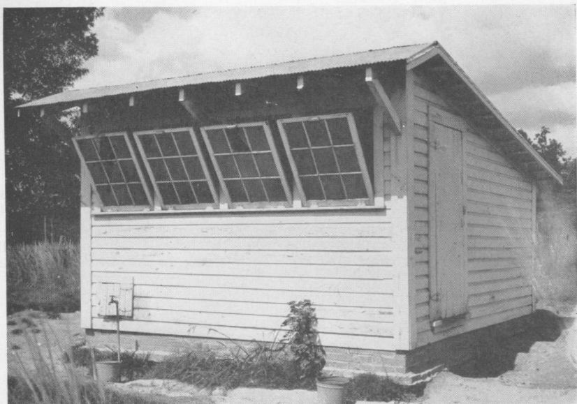
House No. 1. — Solid foundation, wooden floor, and ceiled throughout; windows provide means of controlling ventilation.
