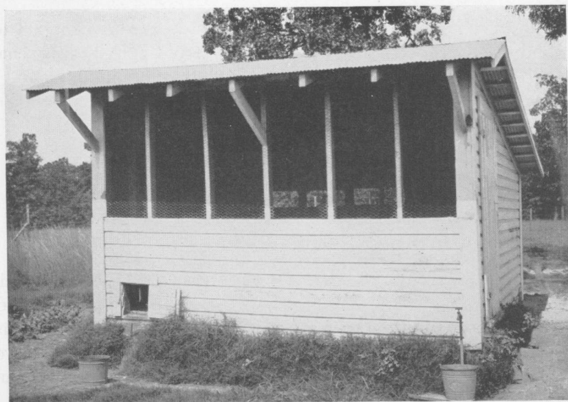
House No. 2. — Solid foundation, wooden floor, no windows, and not ceiled.
