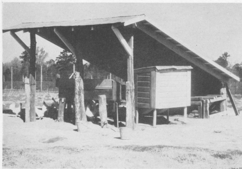
House No. 10. — Roof and low tight north wall.
