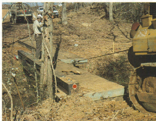
Bridge panels can be installed and removed by a crane or knuckleboom loader (left) or by winching the panels across the stream (right).
