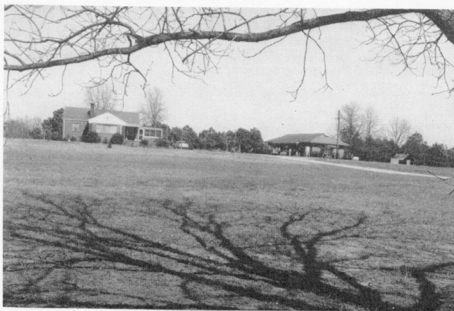
Many meetings and tours for farmers and farm leaders begin here at the headquarters of the Chilton Area Substation.
