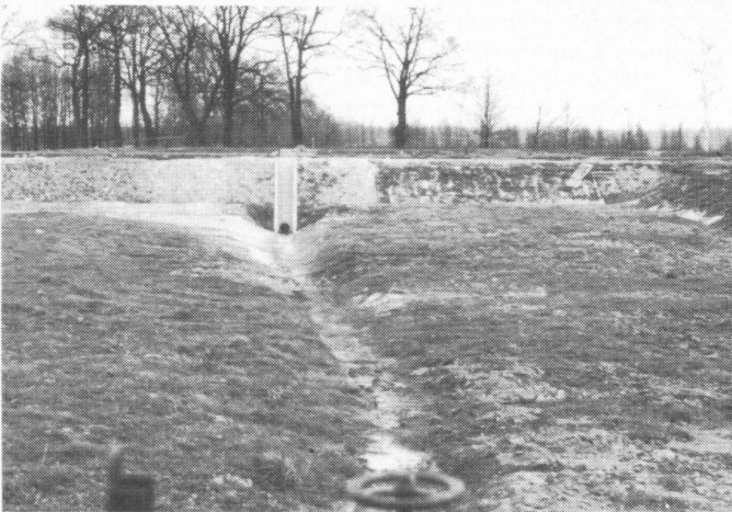
FIG. 2. This 0.5-hectare pond has a ditch down the middle to concentrate fish when drained through the monk at the end. These ponds at the freshwater fishery research stations of the Institute of Zootechnics and the Polish Academy of Sciences are well constructed for fish culture research.
