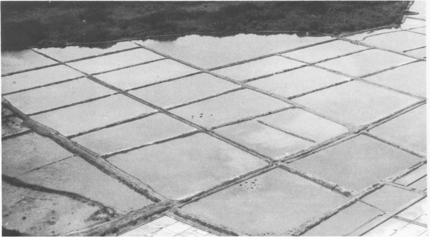
These private salt-drying ponds near Jiquilisco Bay are used to produce salt only during the dry season. With slight modification, however, the 500-hectare pond complex could substantially increase aquacultural production in El Salvador.
