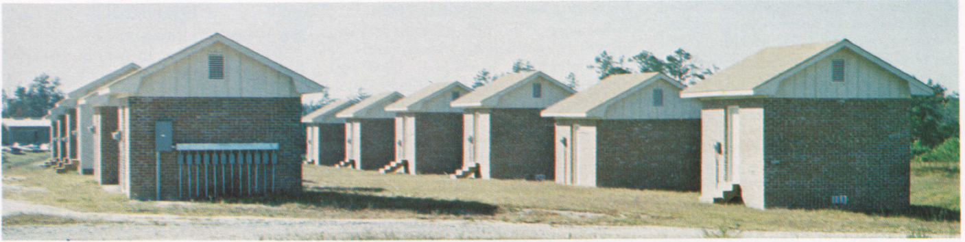
Comparisons of energy requirements for heating and cooling these test houses constructed with different insulation materials and different exterior and interior building materials should provide guides for most energy-efficient homes.
