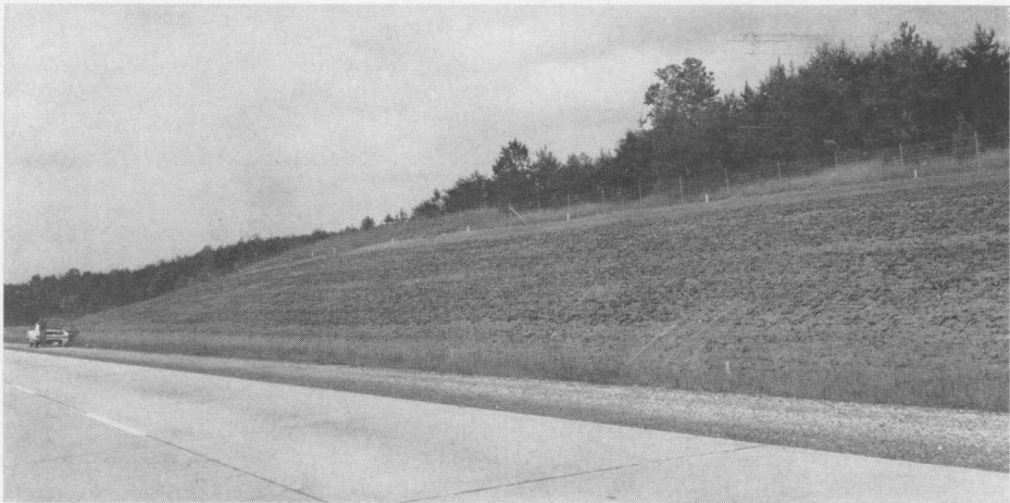
FIG. 2. Highway backslope on I-59 shown ready for planting on May 25, 1966.
