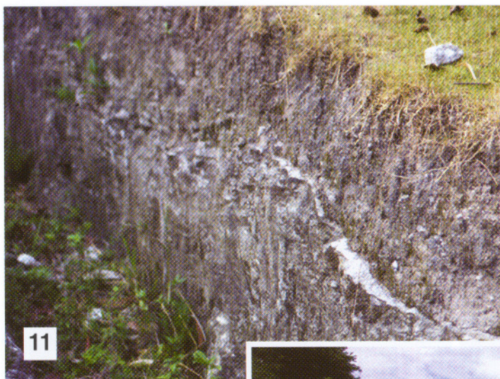
Photo 11. Roadcut at Bergeau, showing petrocalcic horizon at surface of limestone bedrock. This is caused by precipitation of dissolved calcium carbonate onto bedrock, rendering it impervious to water. Petrocalcic horizons were also observed at Pernier and Titanyen.
