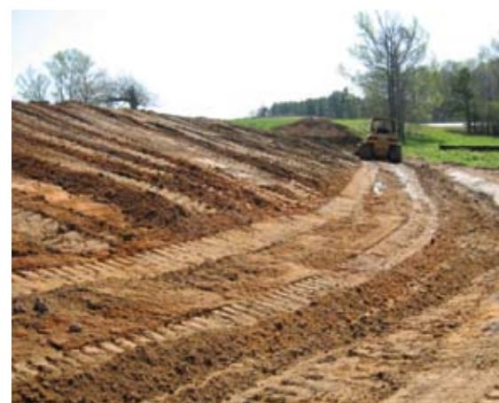
CREATING A SLOPE—Work has begun on a new study area at E.V. Smith Research Center in Shorter to identify ways to better control erosion and water runoff on steep slopes, which will help farmers, road builders and contractors protect soil and water while also developing land.
