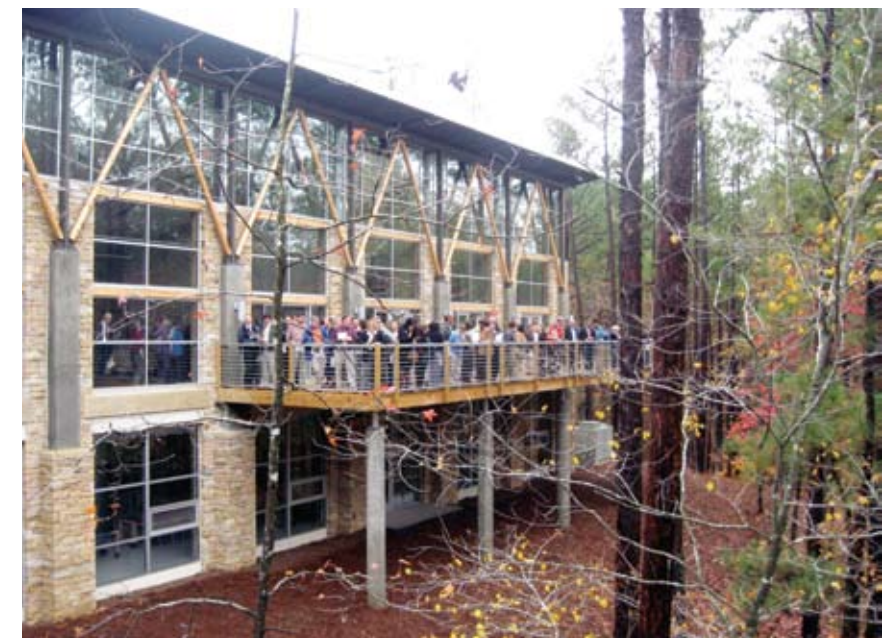
NATURAL CHOICES – The new 17,550-square-foot Alabama 4-H Environmental Science Education Center was dedicated in November. Built to teach as well as demonstrate how to protect our environment, the center is located in a wooded landscape at the Alabama 4-H Camp in Columbiana and is the first planned gold-certified Leadership in Energy and Environmental Design (LEED) environmental education building in Alabama and in the eastern United States.
