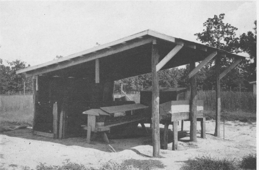
HOUSE NUMBER 4.—Roof and tight north wall.
