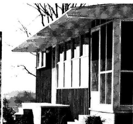
Wide roof overhang shades south wall in summer, exposes it to sun in winter.
