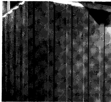
Low-cost board and batten walls give good appearance.
