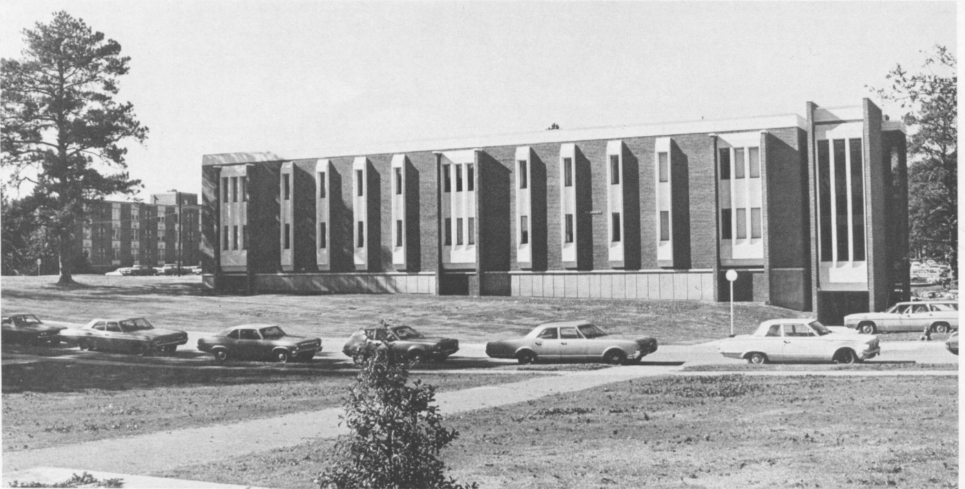
New Fisheries Building at Auburn University.
