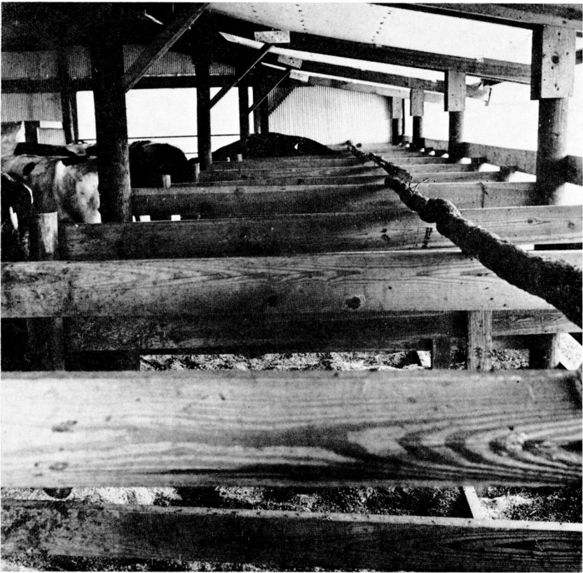
FIG. 3. This view of the free-stall barn at the Gulf Coast Substation shows the neck boards, which were installed 40 inches above the floor.
