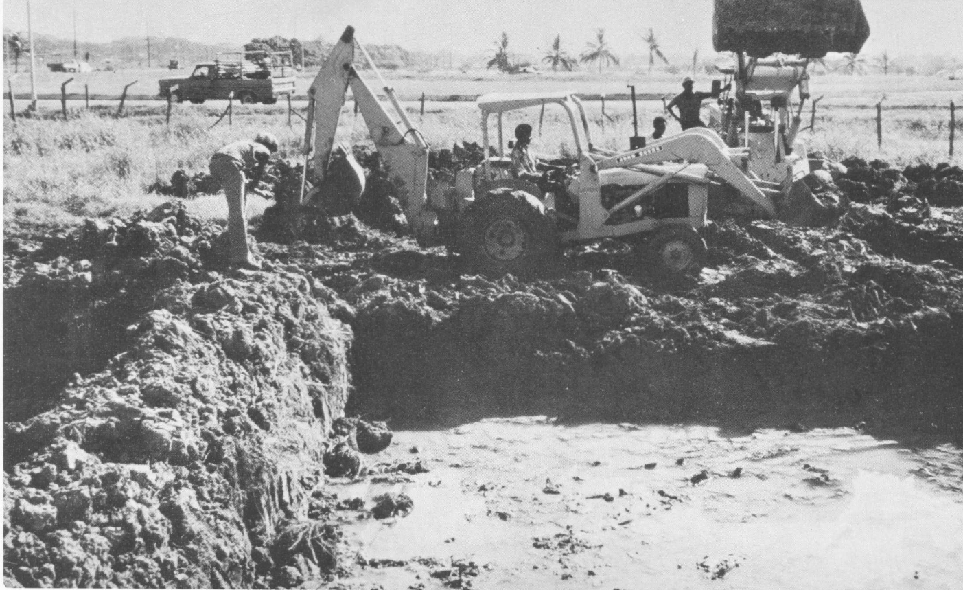
Renovation of fisheries experimental operation at Twickenham Park.
